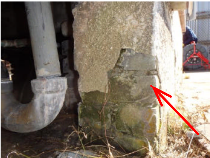
The encapsulation is falling off of some of the piers and can be re-encapsulated (wrapped in a thin coat of cement) to reduce further mortar joint loss.
