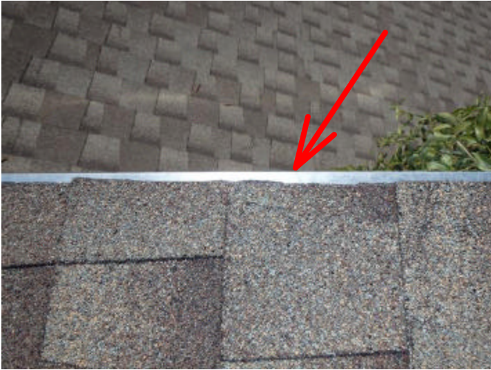
The shingles on the rear of the main roof do not overhang enough, which can cause water to roll back and penetrate the roof sheathing.
