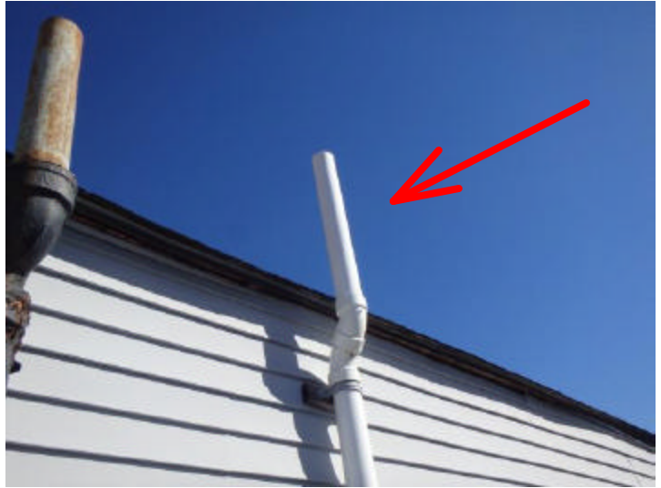
The plastic vent pipes should be painted to prevent damages from the sun's ultraviolet rays.
