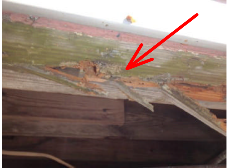
Damages were noted to the rear foundation sill. This deteriorated foundation sill should be replaced to ensure it's structural integrity.
