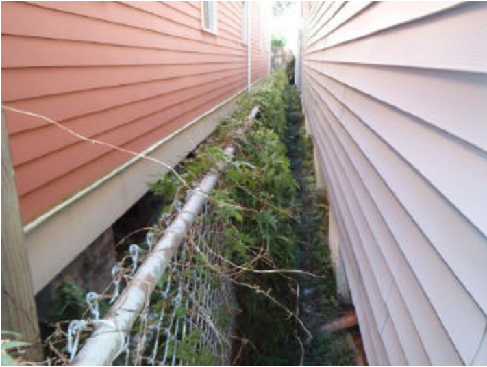
The vine growth on the rear of the house and the fence should be removed to minimize damage potential.
