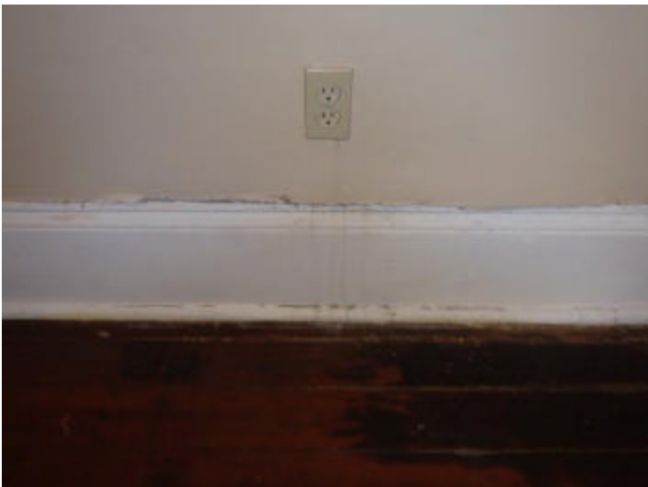
Moisture stains were noted on the floor and baseboard and a loose patch with water stains was noted on the right wall in the 4th bedroom. Damages to the underlying wood, if any, could not be evaluated, due to the finished walls. We recommend further evaluation to determine the source of the leak and repairing as necessary.
