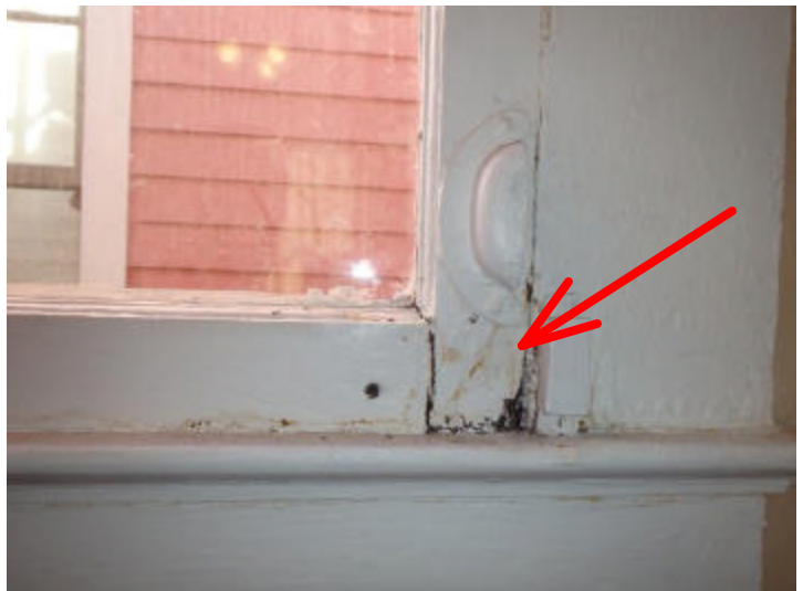
Water stains were noted on the insides of some of the wood windows from moisture penetrations. This condition could be the result of the heavy pane glaze cracking noted on the exterior. We recommend monitoring these stains and repairing as necessary.
