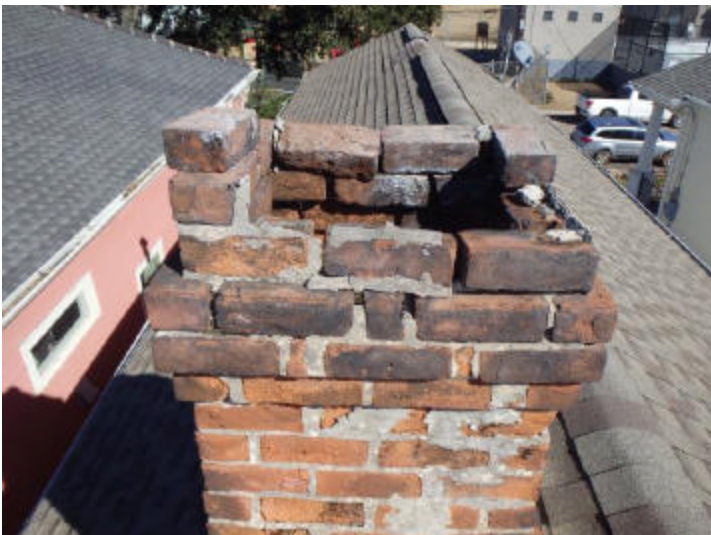
A few loose and missing bricks, which should be replaced, were noted at the chimney on the roof.
