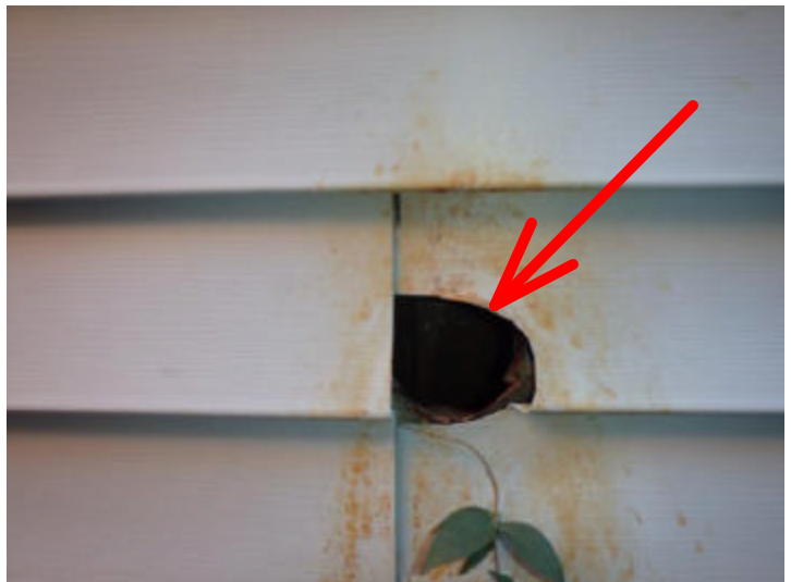
The penetration hole through the exterior siding on the right by the plumbing vent should be sealed to prevent moisture from entering the wall cavities.
