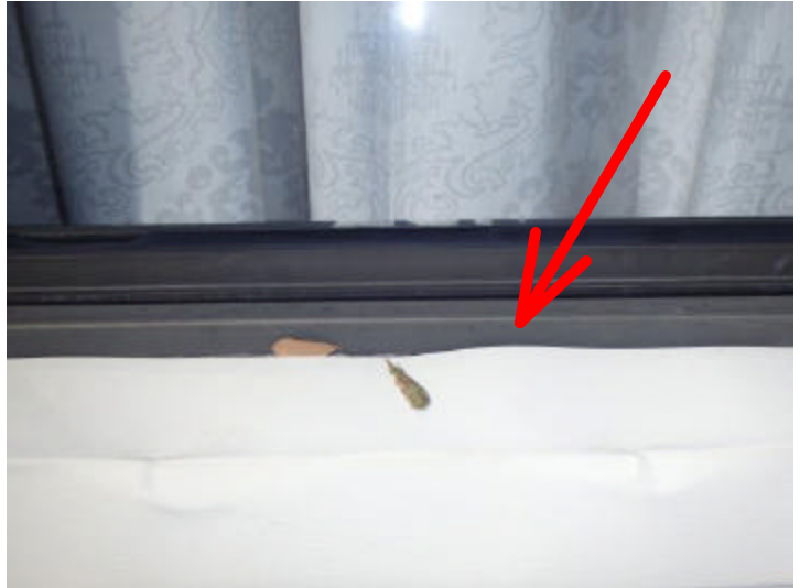
Some of the metal capping at the window sills is wavy and not caulked, which can cause moisture intrusions.
