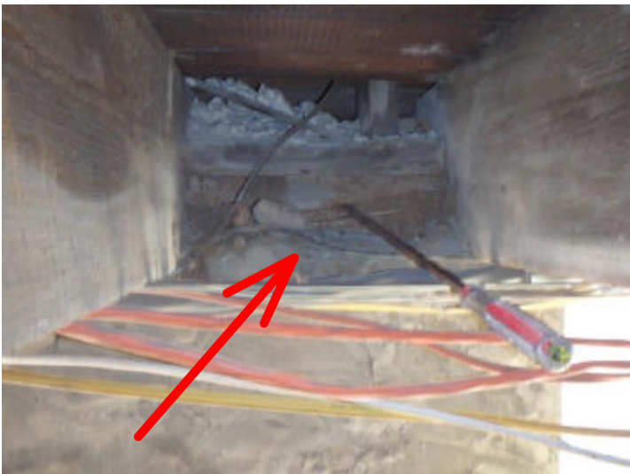
Damages were noted to the foundation sill over the 2nd pier on the left. This deteriorated foundation sill should be replaced to ensure it's structural integrity.
