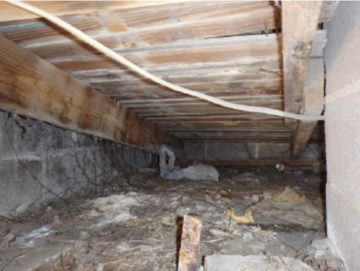
The wood form boards at the front and rear porches can be removed as they are not structural and can promote termite infestations.
