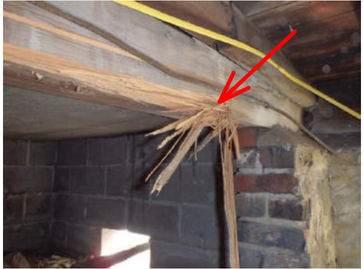
Damages were noted to the front foundation sill. This deteriorated foundation sill should be replaced to ensure it's structural integrity.
