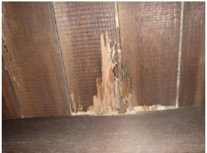
Damages were noted to the tops of the floor joists and to the floor boards in front of the first chimney in the crawlspace, which causes the floors to be loose. The tops of the floor joists can be sistered and the floor boards re-nailed to properly secure them.
