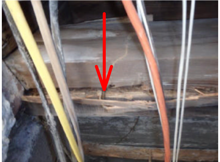
Damages were noted to the cross sill located by the pier to the left side of the 2nd chimney foundation. This deteriorated foundation sill should be replaced to ensure it's structural integrity.
