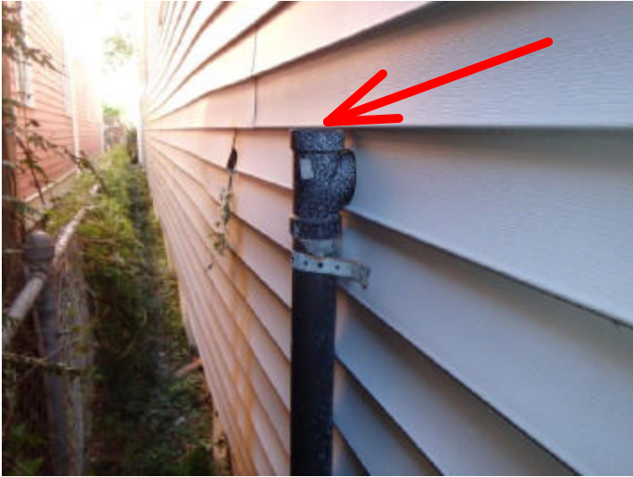
The vent pipe at the right rear should extend above the roof line so that sewer gases can safely escape.
