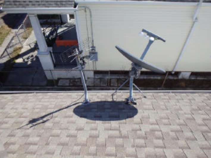
The satellite dish, antennas and brackets on the roof should be removed and the holes sealed to prevent leaks.
