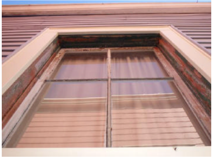
Some of the pane glazing has moderate age cracking and separations, which can cause the window panes to loosen.
