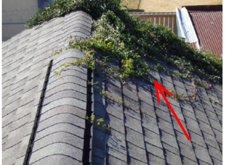
The vines noted on the roof should be removed to minimize damage potential.
