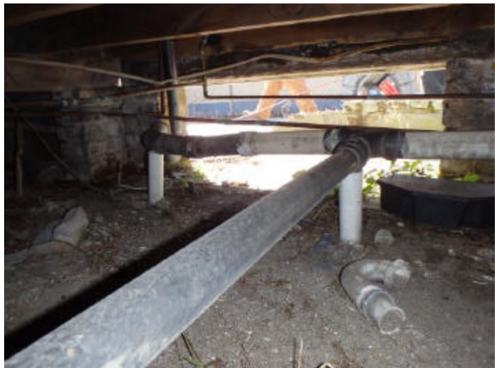
The newer plastic drain lines are improperly supported and are not sloped properly for drainage.
