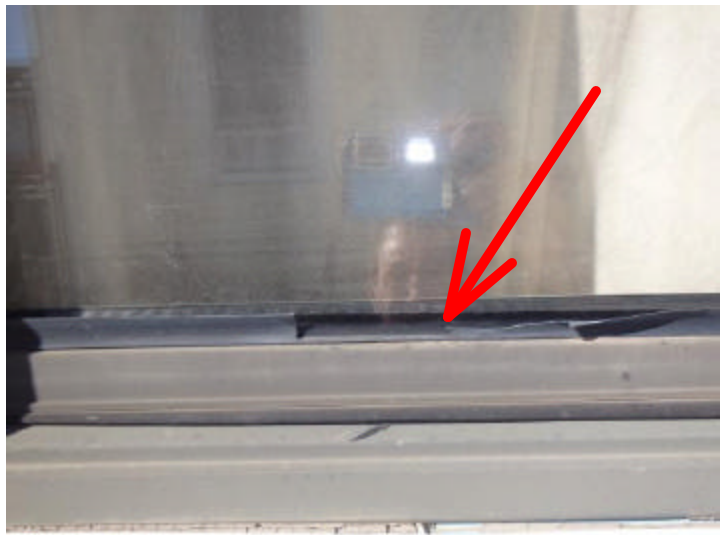
Some of the rubber strips, to secure the window panes to the frame, are cracked.
