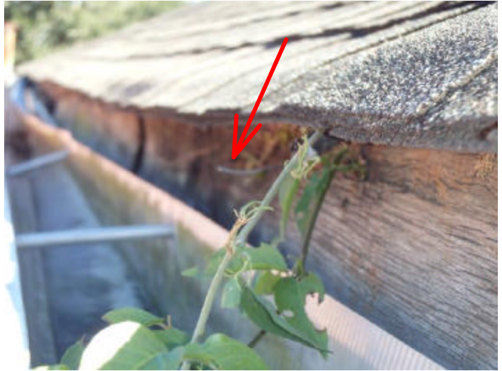
The gutters are falling off of the right side of the house, causing the wood fascia to be exposed.
