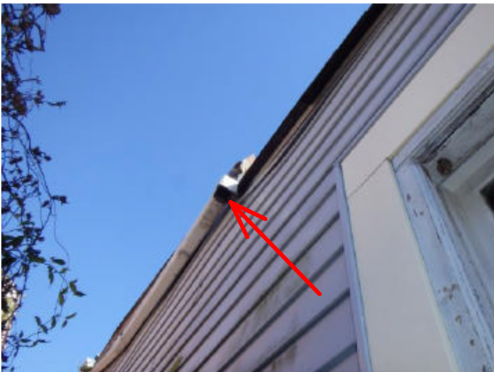
The right rear downspout is missing.
