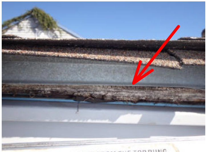
Exposed decking was noted at the rear by the shed type roof. This area should be properly sealed to prevent further moisture damages.
