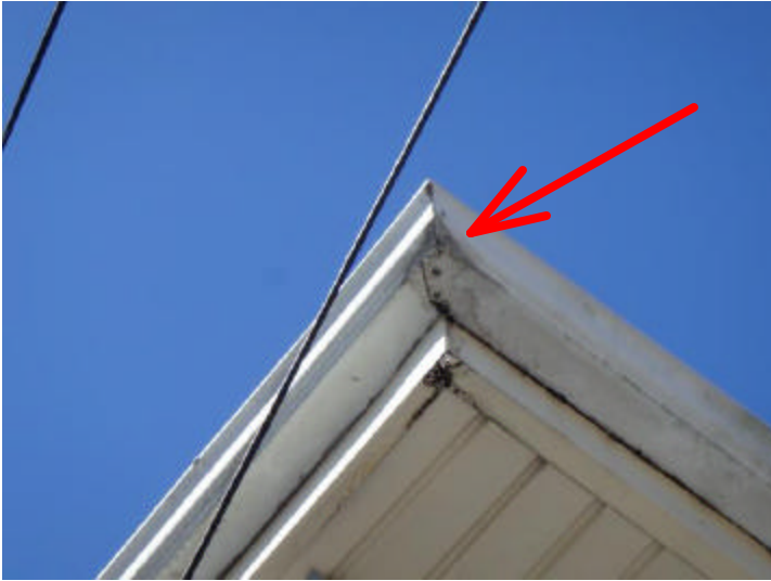
A few of the joints at the gutter runs are leaking.
