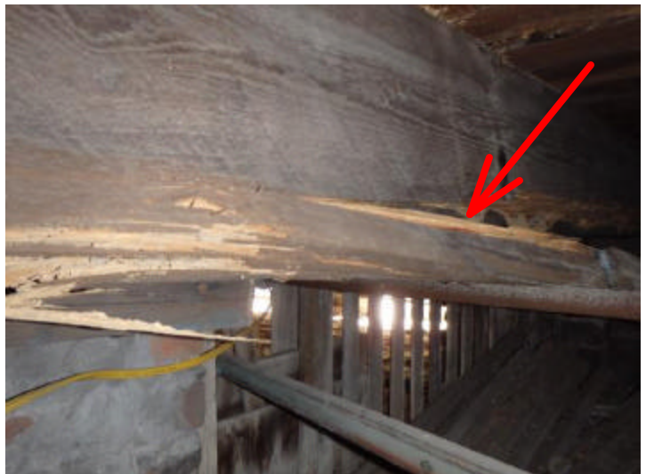
We noted a broken floor joist behind the 2nd chimney foundation. This broken floor joist should be repaired by sistering another board on side of the broken one to ensure it's structural integrity.
