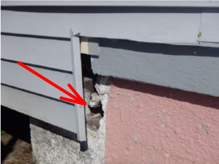
The siding at the rear should be properly sealed to prevent moisture intrusions.
