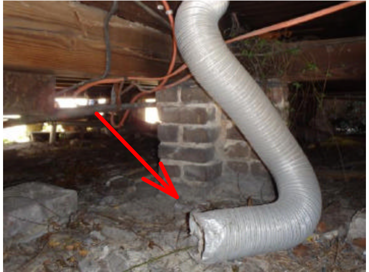
The clothes dryer vents into the crawlspace, which will lead to lint and moisture accumulation. We recommend that the vent pipe be extended to the outside.
