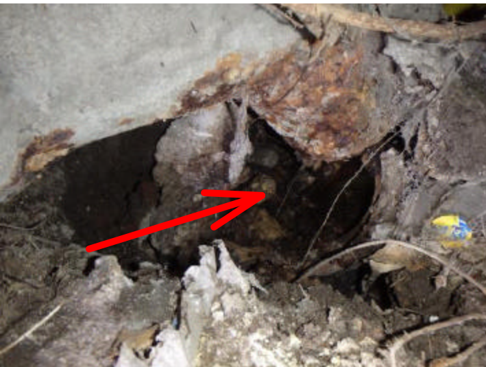
A broken cast iron drain line was noted above ground and underground at the right rear. Please see HyTech Plumbing's separate report for additional details.
