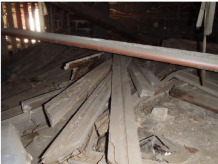
Debris was noted in the crawlspace. This debris should be removed to prevent possible termite infestations and to safely crawl for inspections and service work.
