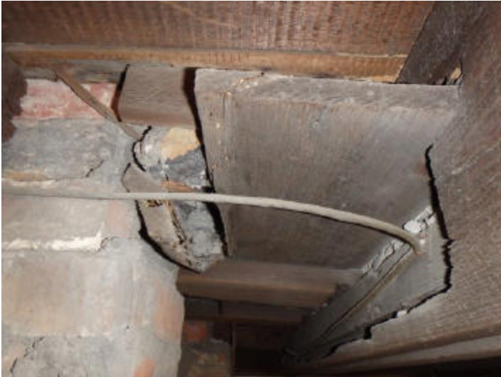
Damages were noted to the blocking at the 2nd chimney foundation. This condition has caused a couple of the floor joists to loosen. These joists should be properly secured to ensure their structural integrity.
