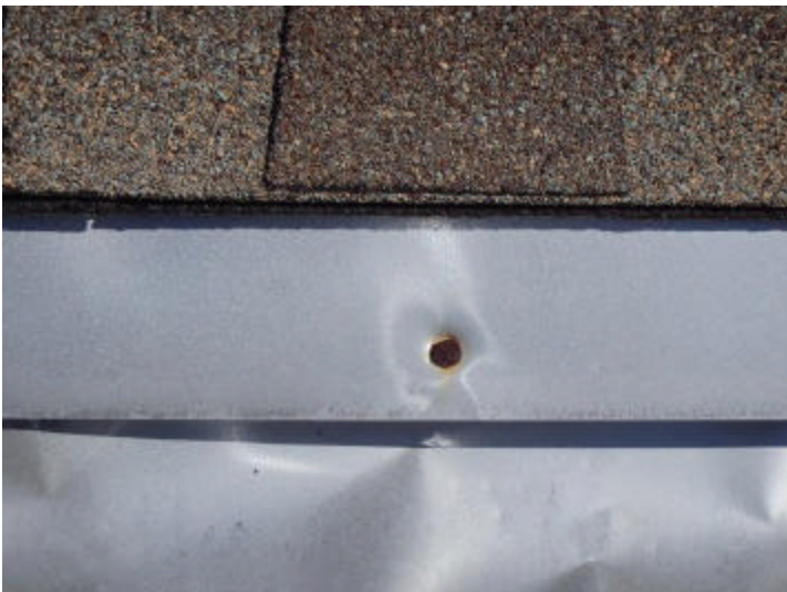
The flashing at the rear of the main house is loose and has exposed and rusted nails.
