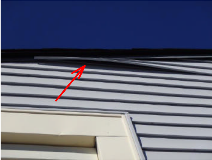
The siding is loose and wavy in various areas throughout.
